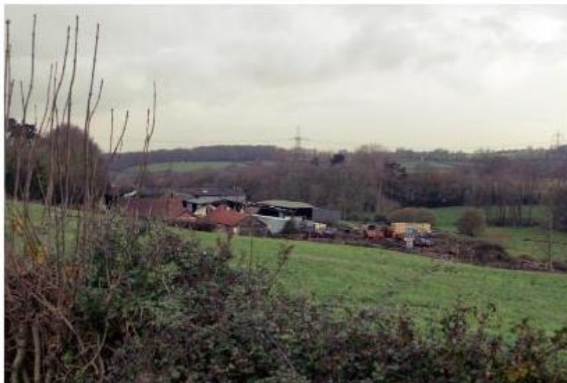
View south from Botley Road - large agricultural buildings fit their rural context due to fragmented roof forms
